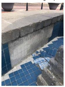
When the fire pits are installed each winter, their weight has caused the tiles in the fountain to chip and break, particularly around the two drains. This winter, whole sheets of tile fell off of the sides of the fountain walls.
